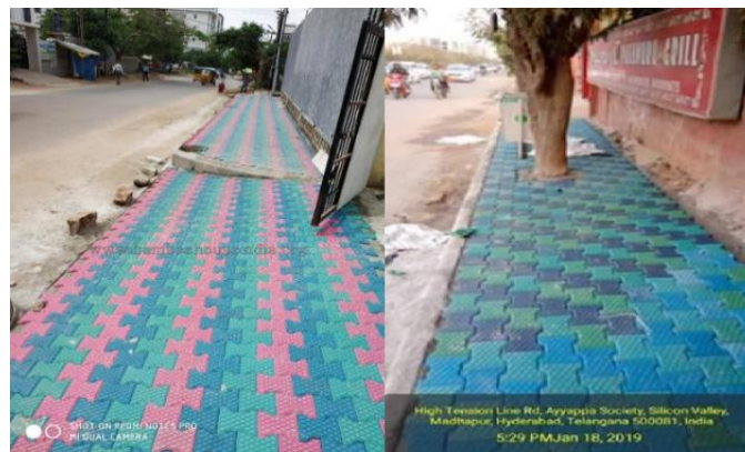
Figure 5: Tiles from waste plastic installed by Municipal Corporation, Hyderabad
